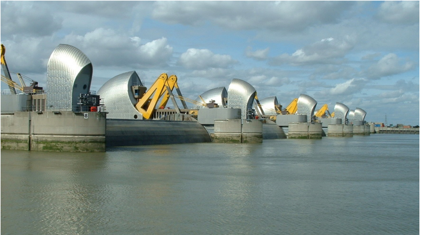
Image 1. A movable system, the Thames Barrier on the Thames River in London, England, was made to stop the surrounding areas from being flooded because of high water levels. Photo: Andy Roberts/Wikimedia Commons
